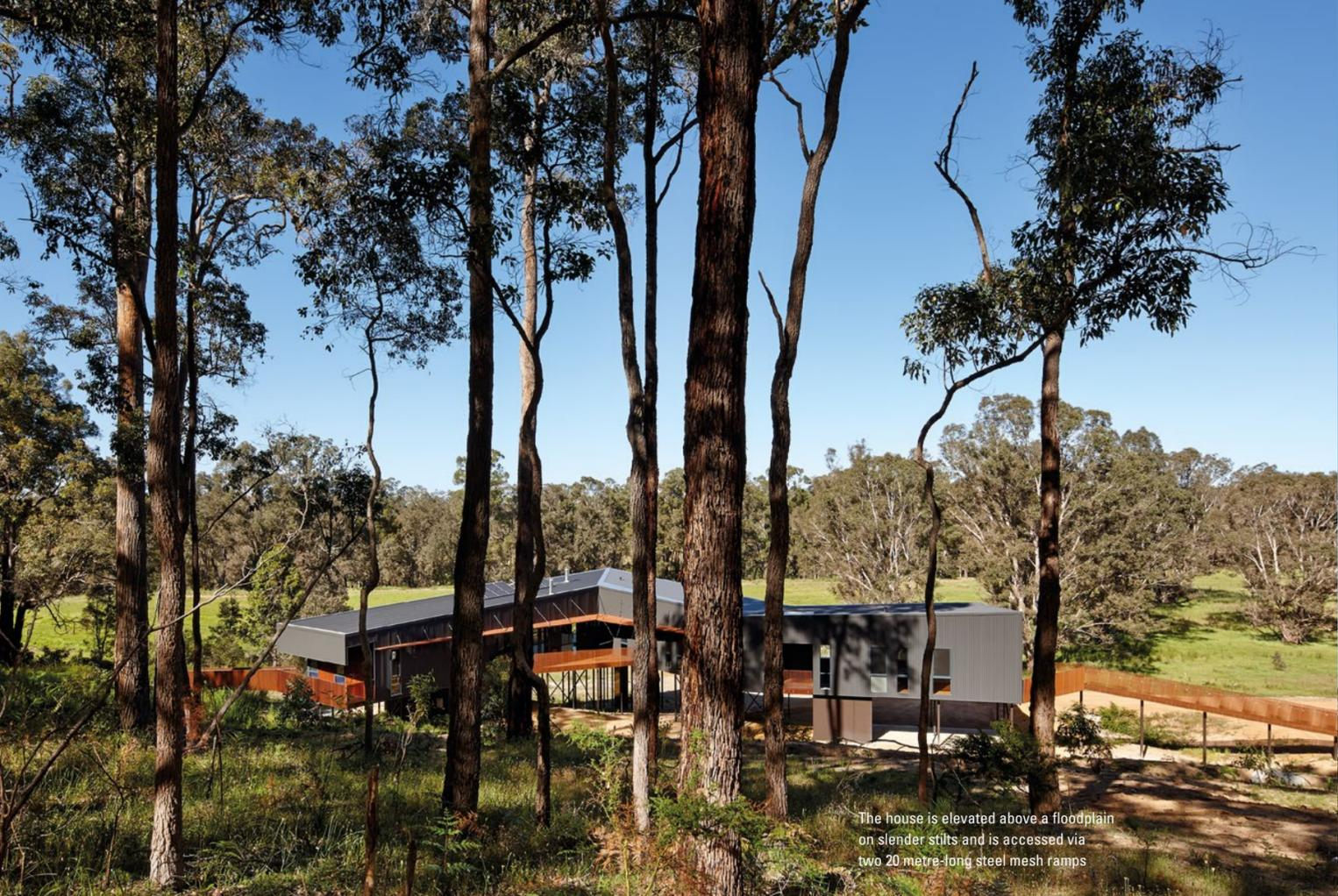
The house is elevated above a floodplain on slender stilts and is accessed via two 20 metre-long steel mesh ramps
