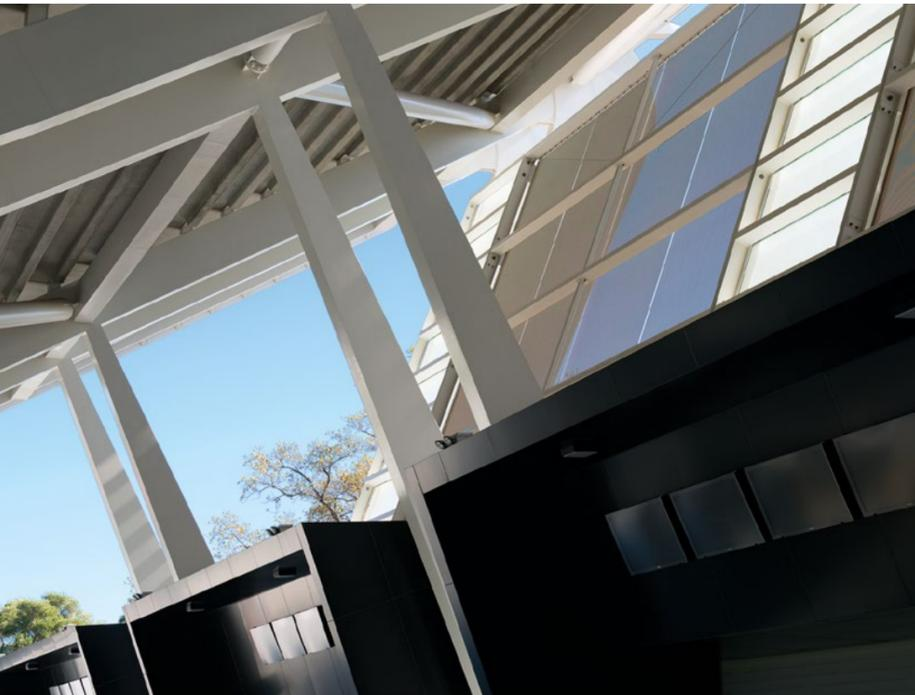
ABOVE: Woven metal mesh is stretched between each of the skeletal frames, allowing natural light to penetrate while protecting the concourse from wind and rain
