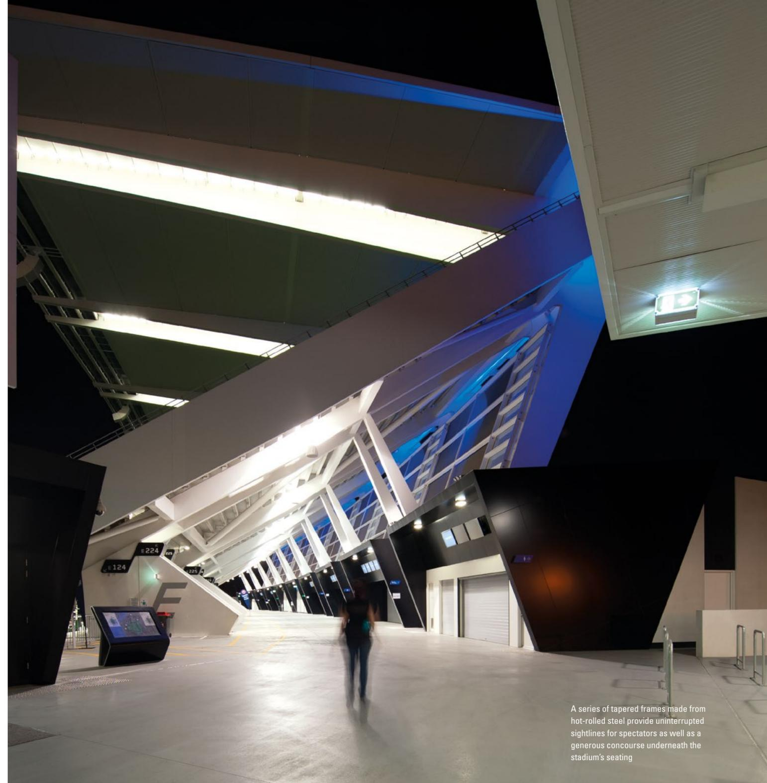
A series of tapered frames made from hot-rolled steel provide uninterrupted sightlines for spectators as well as a generous concourse underneath the stadium's seating
