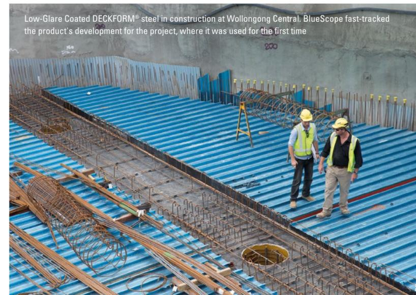
Low-Glare Coated DECKFORM® steel in construction at Wollongong Central. BlueScope fast-tracked the product's development for the project, where it was used for the first time
