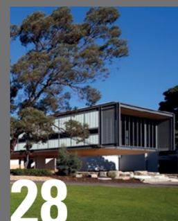
A clever box frame modelled around a Vierendeel truss demonstrates – in the form of two new school pavilions – that faith in engineering and architecture can push the boundaries of possibility
