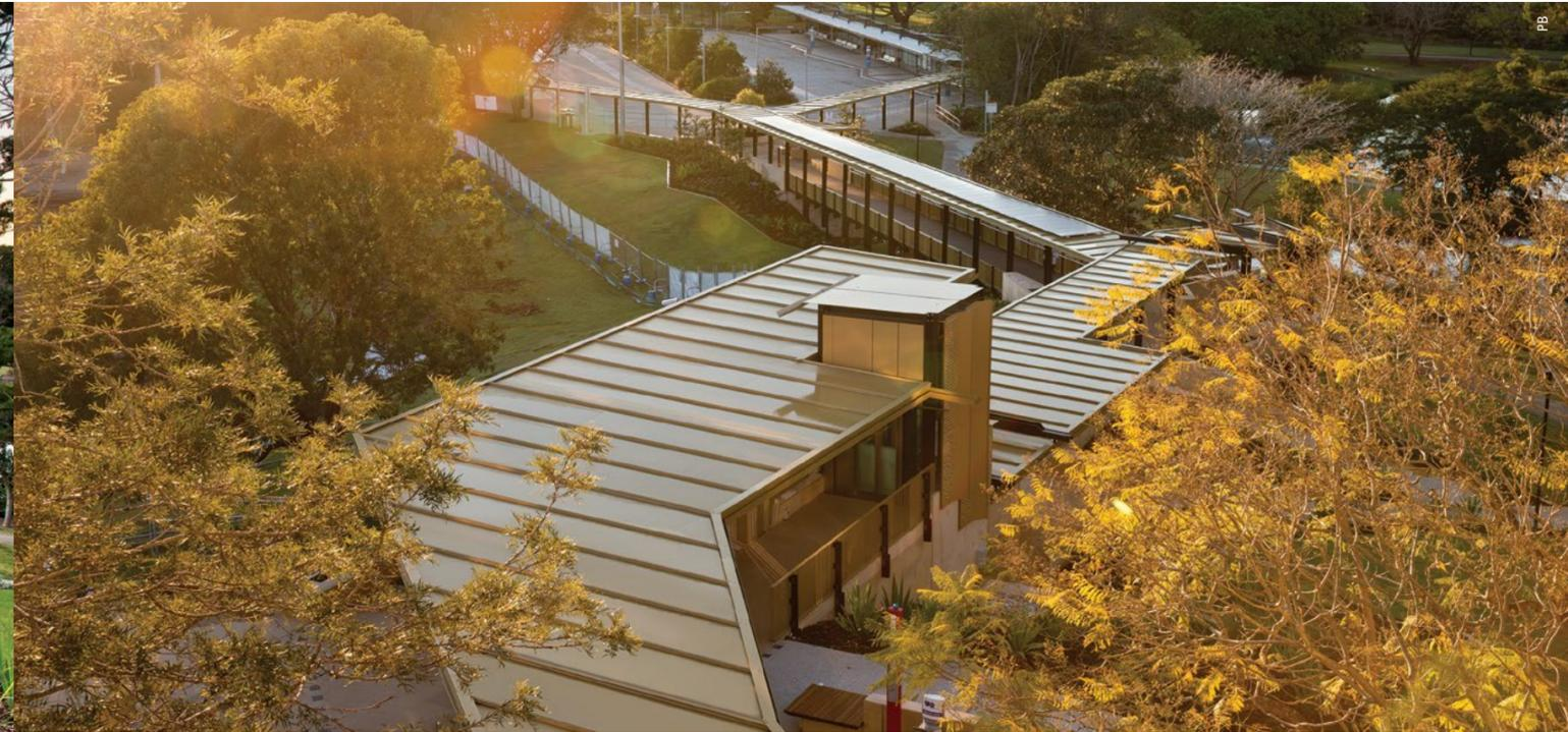
with a cantilevered structure such as this to ensure vibration limits for pedestrian movements and serviceability deflections were not a problem. Also, detailing the pre-cambers to ensure everything looked straight and true was interesting.”
